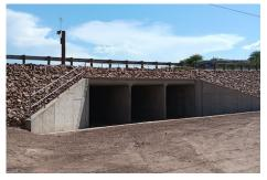
The burn scar left behind by the 2020 Bighorn Fire left some neighborhoods in the Catalina Foothills far more vulnerable to flash floods. In response, Pima County decided to replace the culvert at Finger Rock Wash to increase its capacity and reduce the risk of catastrophic flooding in fireimpacted areas. With the reopening of Skyline Drive on Aug. 31, the project is officially complete
