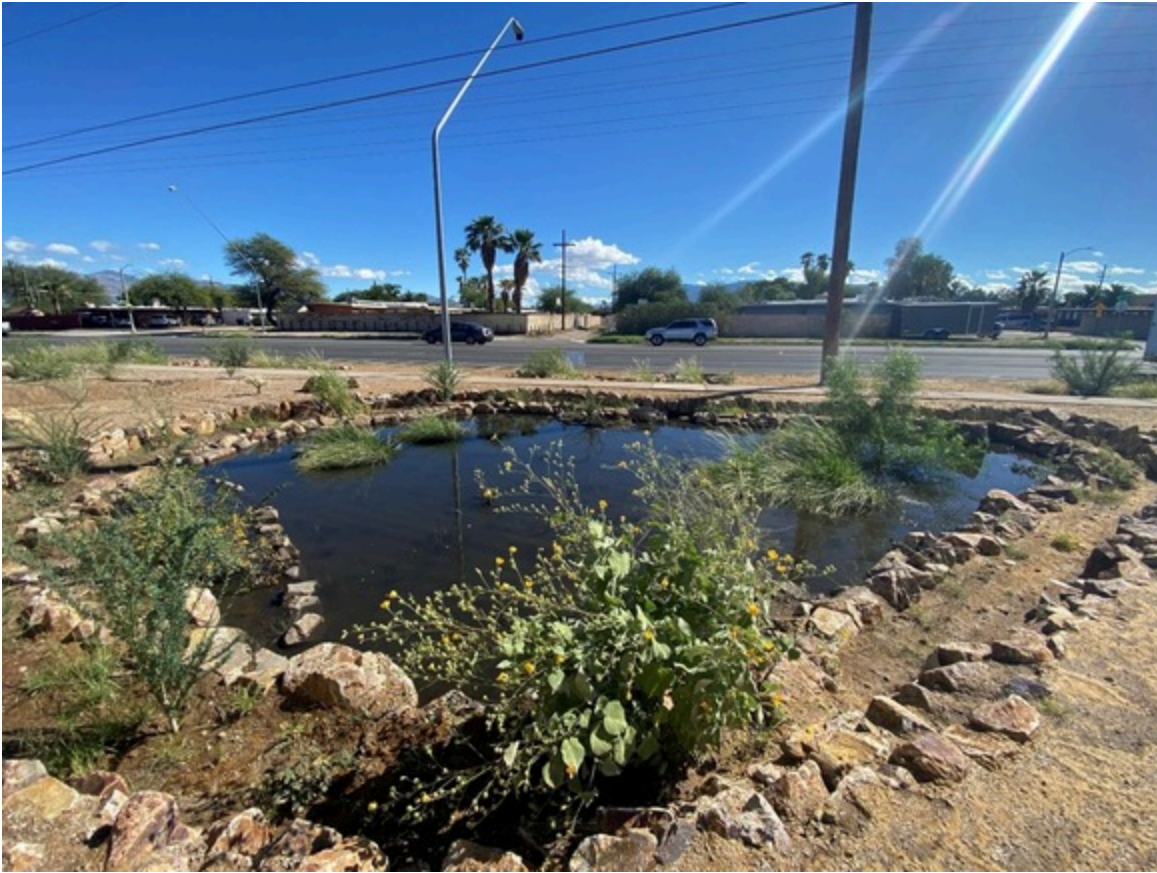
Green stormwater infrastructure project on Pantano, installed by Storm to Shade
